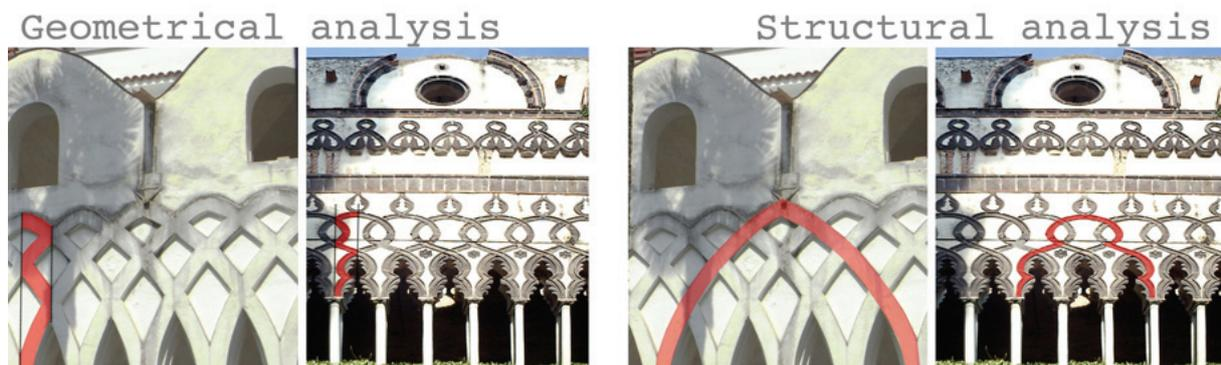
Fig. 2: the Cathedral of Amalfi and Villa Rufolo (Ravello). Geometrical and structural analyses.
