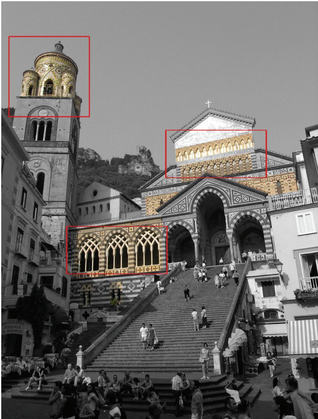
Fig.1: the Cathedral of Amalfi. Highlight of the interwoven arches of the façade and of the bell tower.
