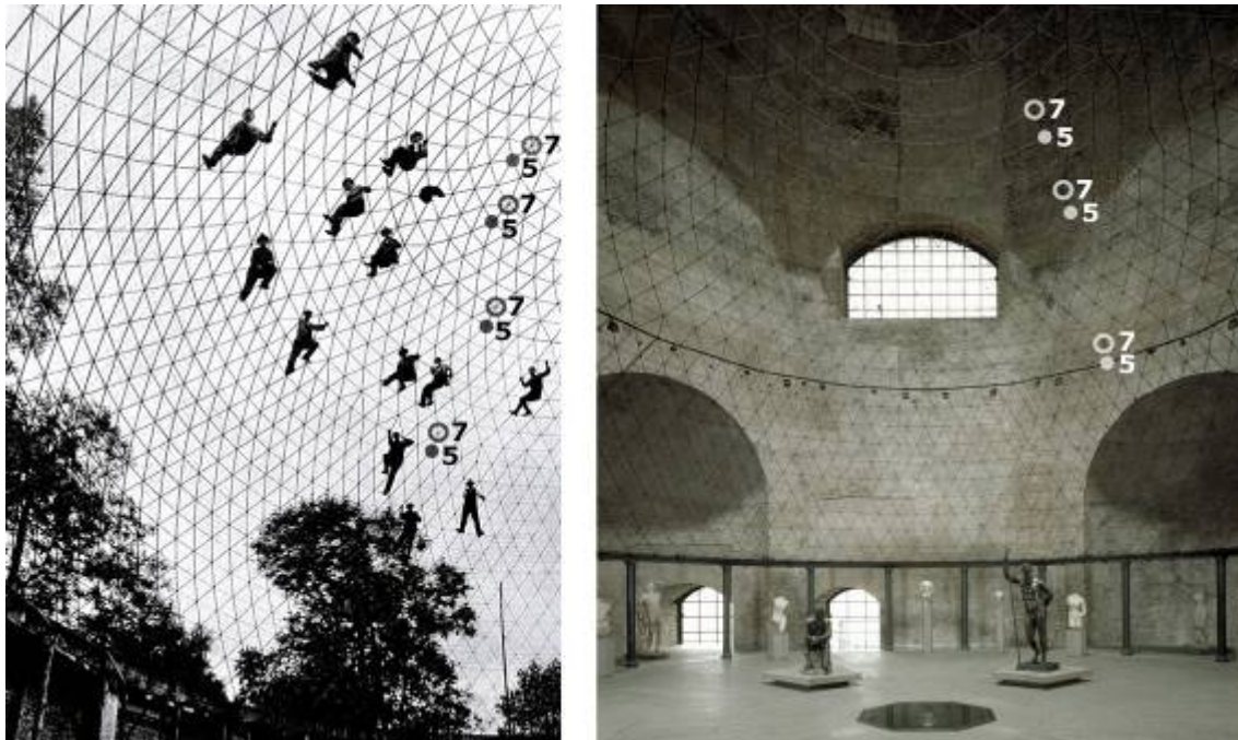
Figure 3. Planetarium Jena (historical photo from Greco C., Le prime cupole in cemento armato sottile , 1997, p.298) and Planetarium in Rome (photo by Casabella, 1998, n. 654, March). In the photos we indicate vertices of degree 7 and vertices of degree 5.
