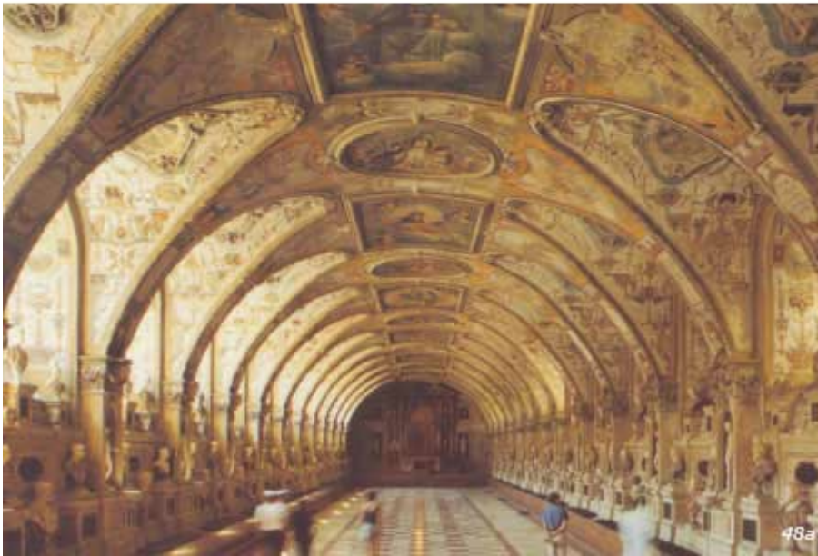
Fig. 7.48 In architecture, vaults often feature interesting intersection curves (including parts of conic sections). (a) Intersection curves in the barrel vault of the Residenz (1569–1571) in Munich. (b) A cross vault in a building entrance (image courtesy of Martin Reis). (c) Model of a vault.
