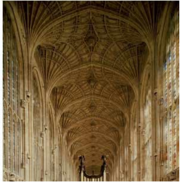
Fig. 7.33 Parameter lines support the spatial impression of surfaces. (a) The same surface with and without parameter lines. (b) The usage of parameter lines in architecture is illustrated by means of the fan vault of the King's College Chapel (1446–1515) in Cambridge.
